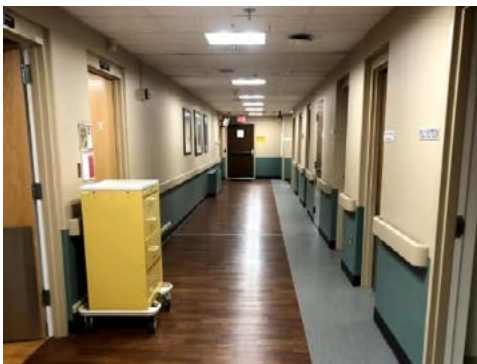
Western half of main east-west hallways
